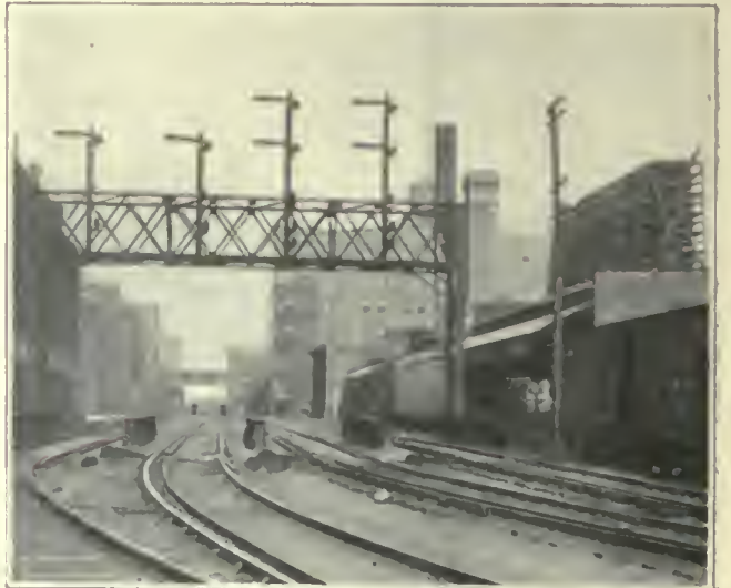
FIG. 289. SIGNALS. Signal bridge on the St. Charles Air Line near Clark Street.
